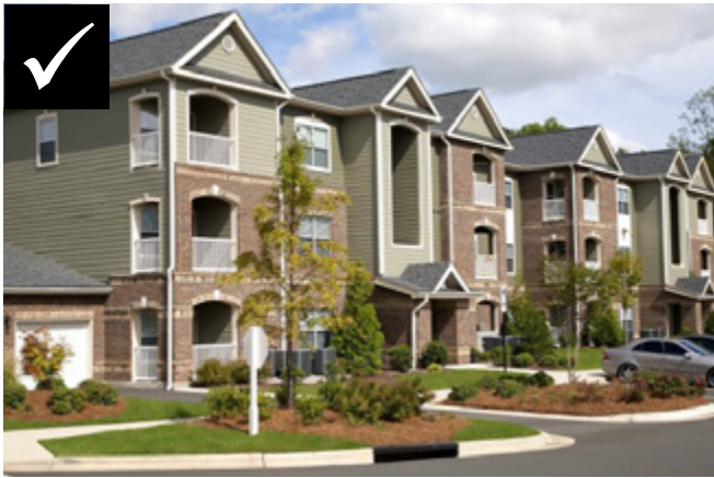
Facade articulation with recesses and projections
