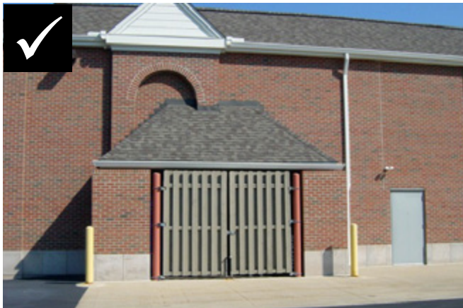
Screened ground-level equipment
