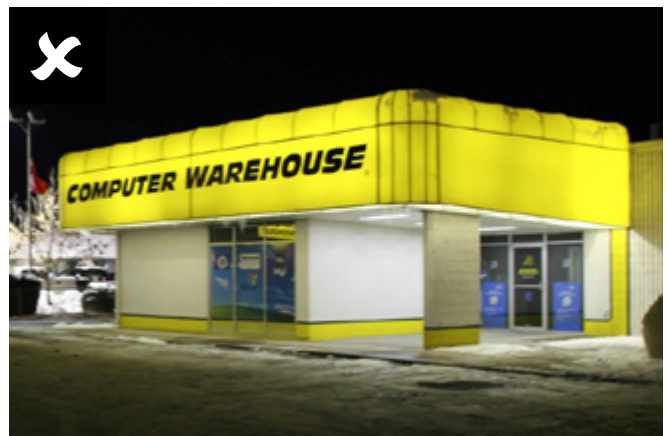
Backlit awning spanning building length
