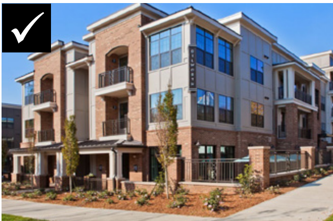
Flat roof with decorative parapet and variation
