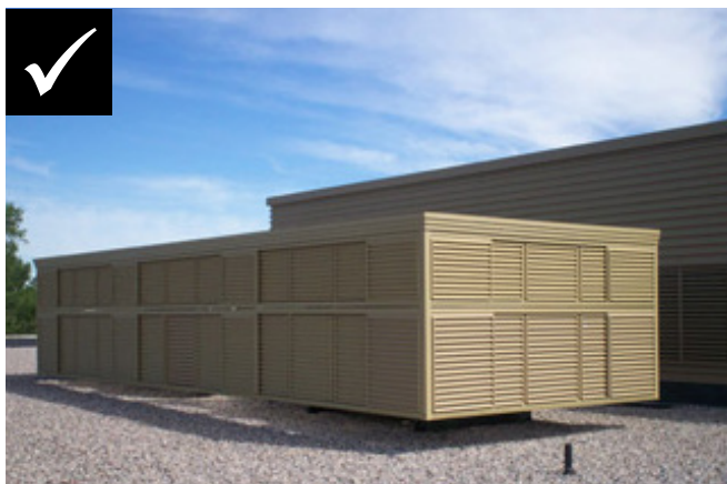
Screened roof-top equipment
