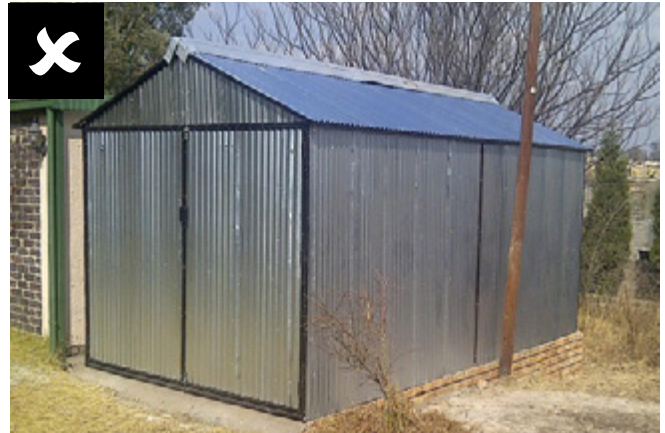
Materials do not match principal structure
