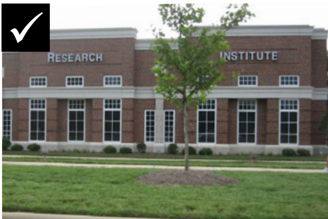
Continuous parapet with height changes
