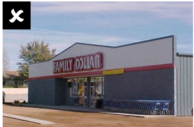
Painted concrete block and metal facades
