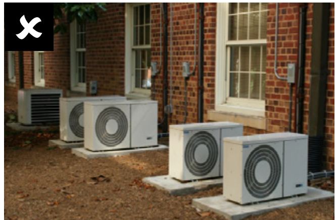
Unshielded ground-level equipment
