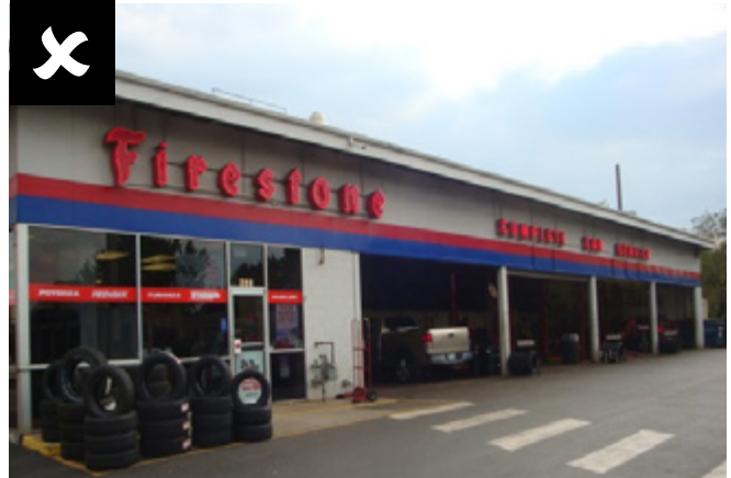
Service bays on primary facade
