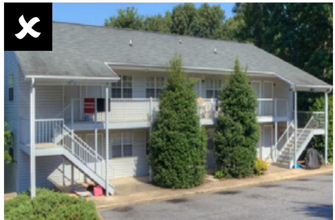
Exterior stairs and circulation corridors
