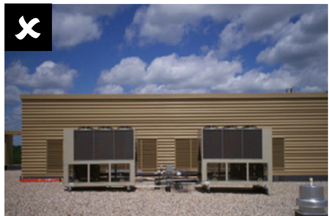
Unshielded roof-top equipment
