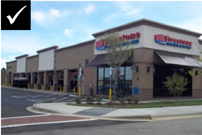
Service bays on secondary building wall
