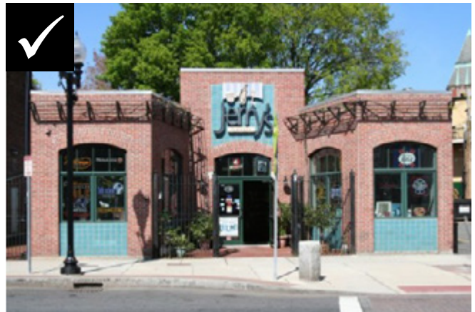
Recessed openings and decorative metalwork
