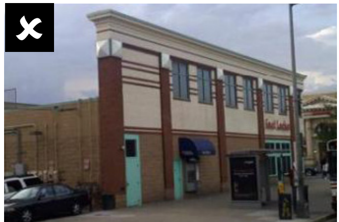
Non-continuous parapet without height changes
