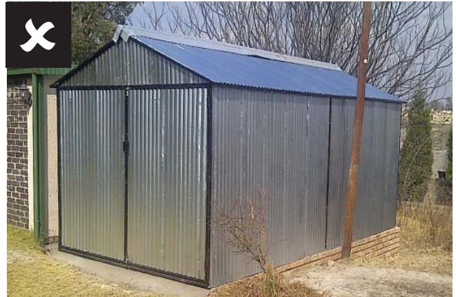
Materials do not match principal structure
