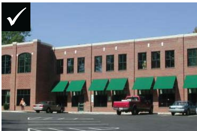
Awnings over windows
