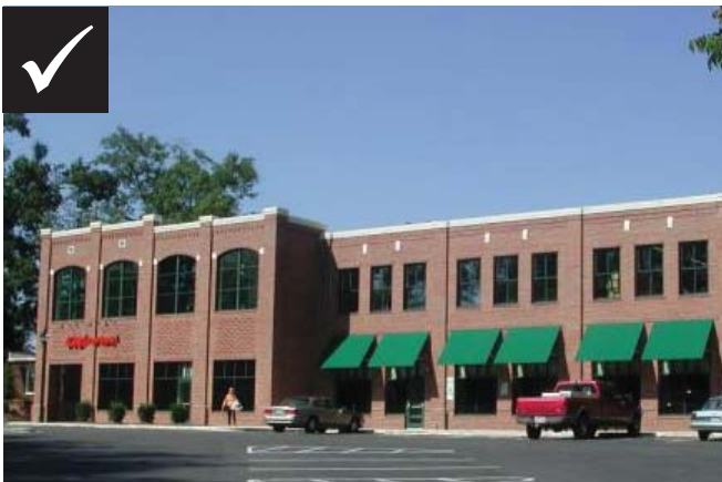
Awnings over windows
