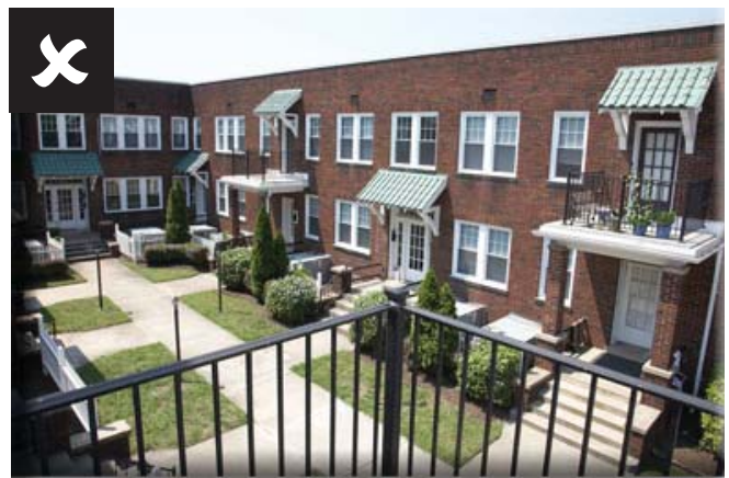
Flat roof with no decorative parapet or variation
