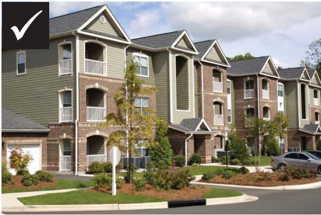
Facade articulation with recesses and projections
