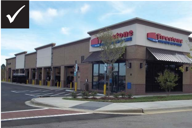
Service bays on secondary building wall
