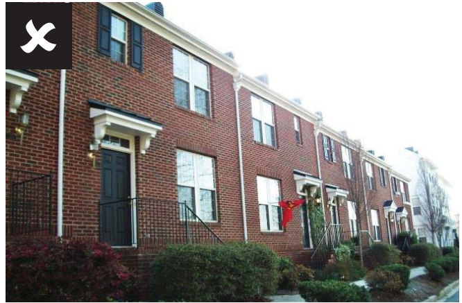
No facade articulation
