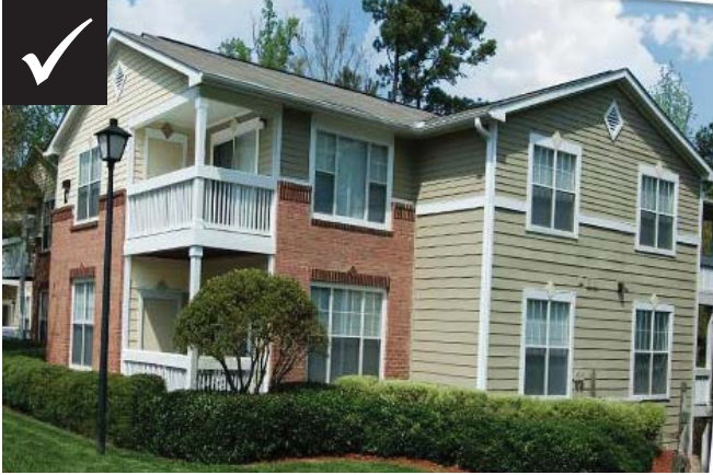
Adequate windows with regular rhythm and alignment
